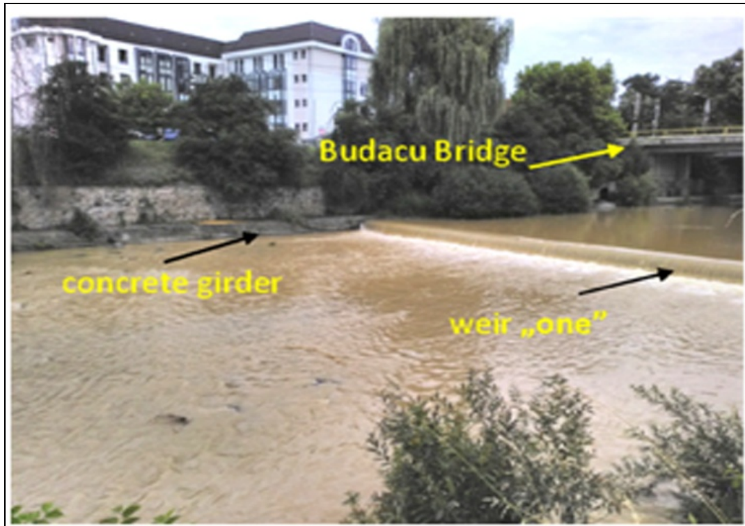
Figure 1a: weir image from the left river bank.
